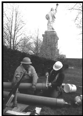
Trim spigot end before attaching pulling eye.
