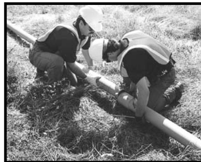
Attach the next piece of Bore-Gard.
