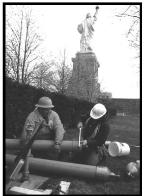
Trim spigot end before attaching pulling eye.
