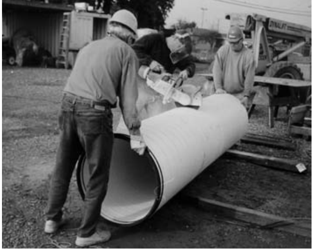
Cutting pipe to length
