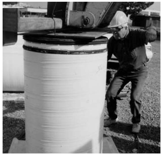
Field inserting gasketed ring
