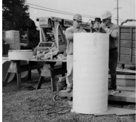
Routing in vertical position
