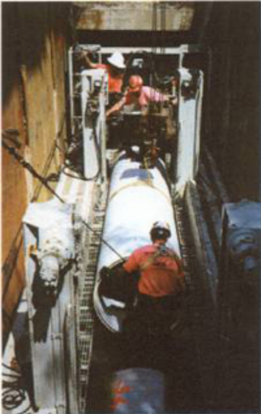
A special sliplining push unit with power for up to 200 tons thrust is employed on the project.
