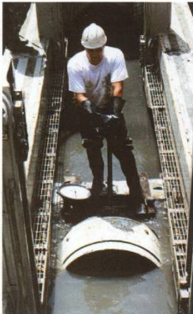
A crew member follows a short coupling section as it moves to join the pipe string.
