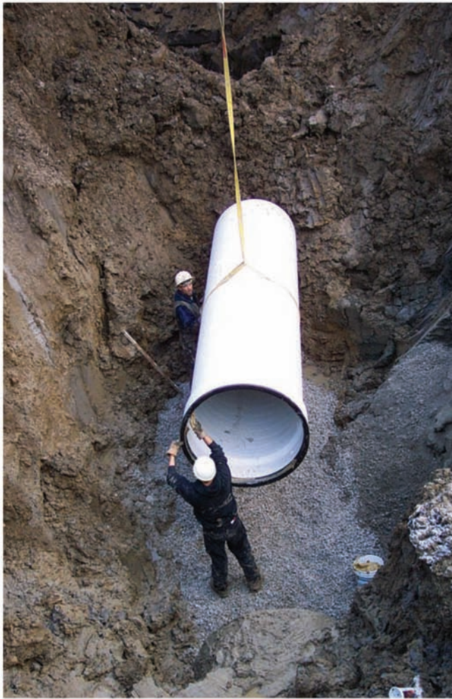
Bedding was critical to pipe placement. The triple gasket can be seen on this pipe segment.
